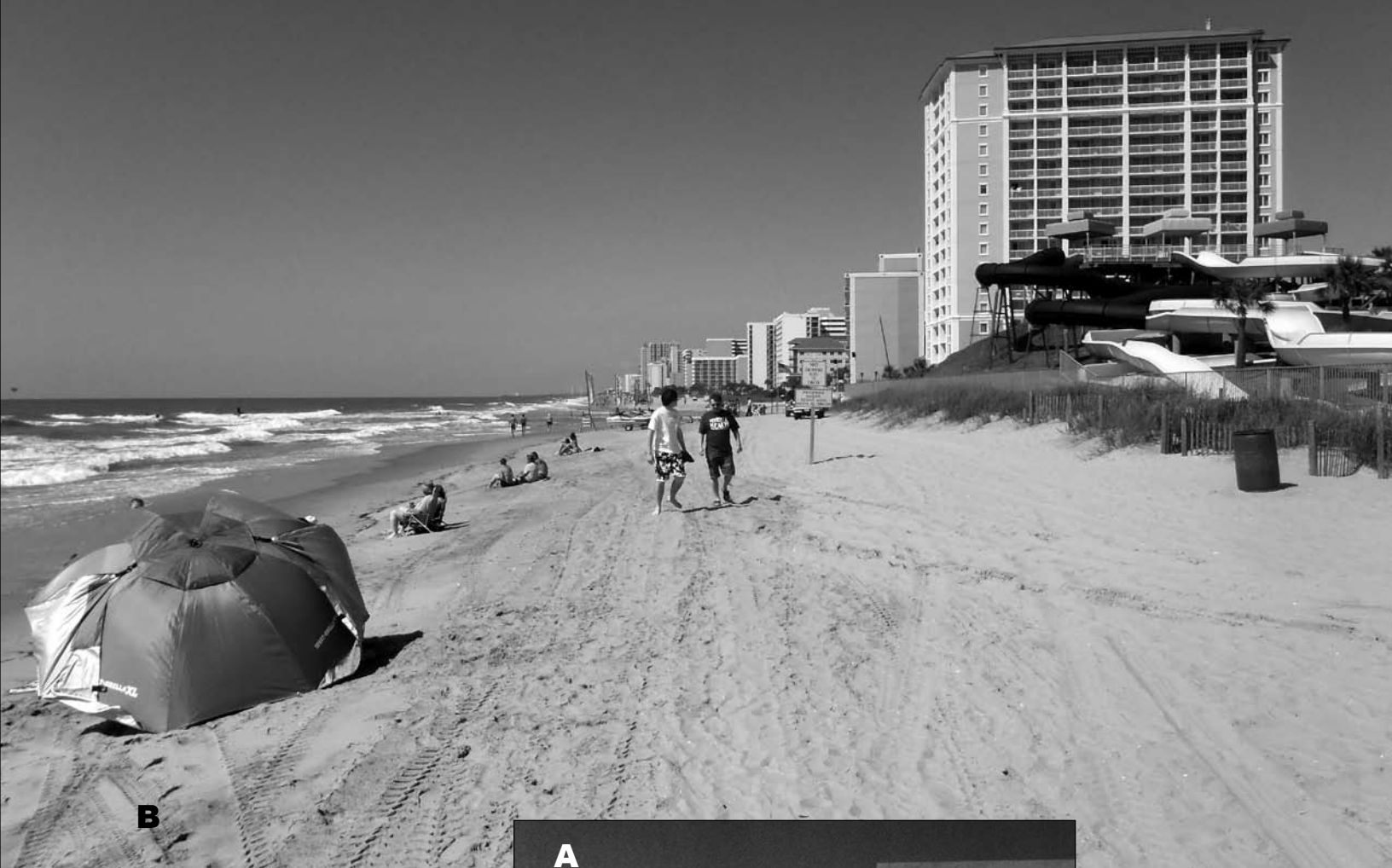
Figure 8. High-tide conditions in Myrtle Beach (2nd Avenue South) prior to nourishment (A — 1986) and after four events (B — 2012). The concrete seawall protecting “Wild Rapids” Water Park in 1985 is now buried and fronted by ~75 ft of vegetated dunes and dry-sand beach.
