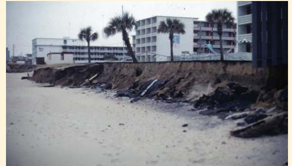
17th Avenue South (1983)
