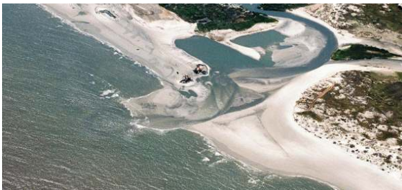
Excavating a tidal inlet through an incipient barrier spit
