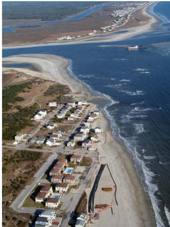
FIGURE 25. Severe, localized erosion adjacent to a tidal inlet (Ocean Isle Beach, NC). Net longshore transport is into the inlet. A terminal groin positioned downdrift of these houses (ie – middle of photo) is probably the most cost-effective way to hold the beach in place with a secondary benefit of reducing shoaling in the channel. Once filled to capacity, properly designed groins will bypass excess sediment.
