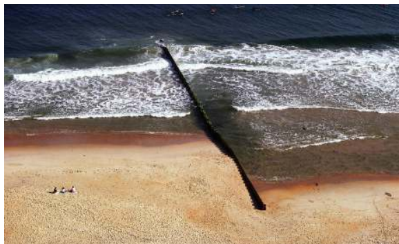
Cape Hatteras (NC) groin – trapping sand moving from left to right (N to S).
