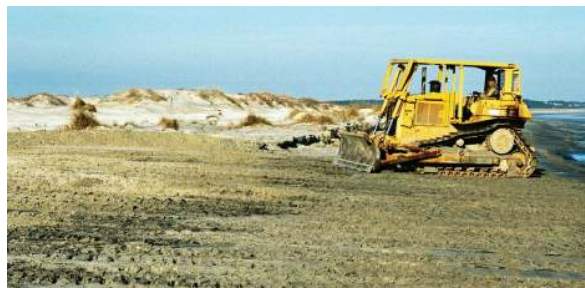
Beach scraping via bulldozer
