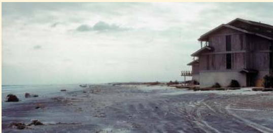
Post Hugo washover beach – note negligible damage to building.
