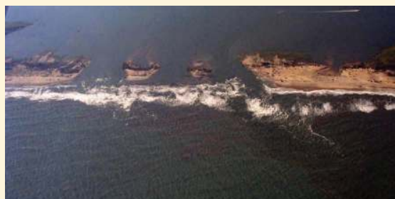
Storm breach – Hatteras Island (NC) – 2003
