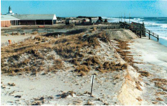
Isolated shore protection structures (such as this bulkhead along the New York coast) locally modify erosion rates but do not alter the regional erosion trend. [Photo by M Kana]
