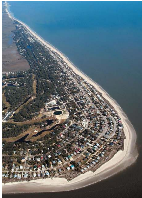
Edisto Beach (SC) – Net longshore transport is from top to bottom and “into the bight” along this barrier spit. Scalloped vegetation line marks locations of groins buried by a recent nourishment project. [Source: CSE]
