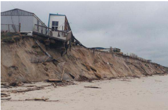
Indian Beach – Bogue Banks (NC) – after Hurricane Floyd (1999) – top of escarpment is >20 ft above MSL
