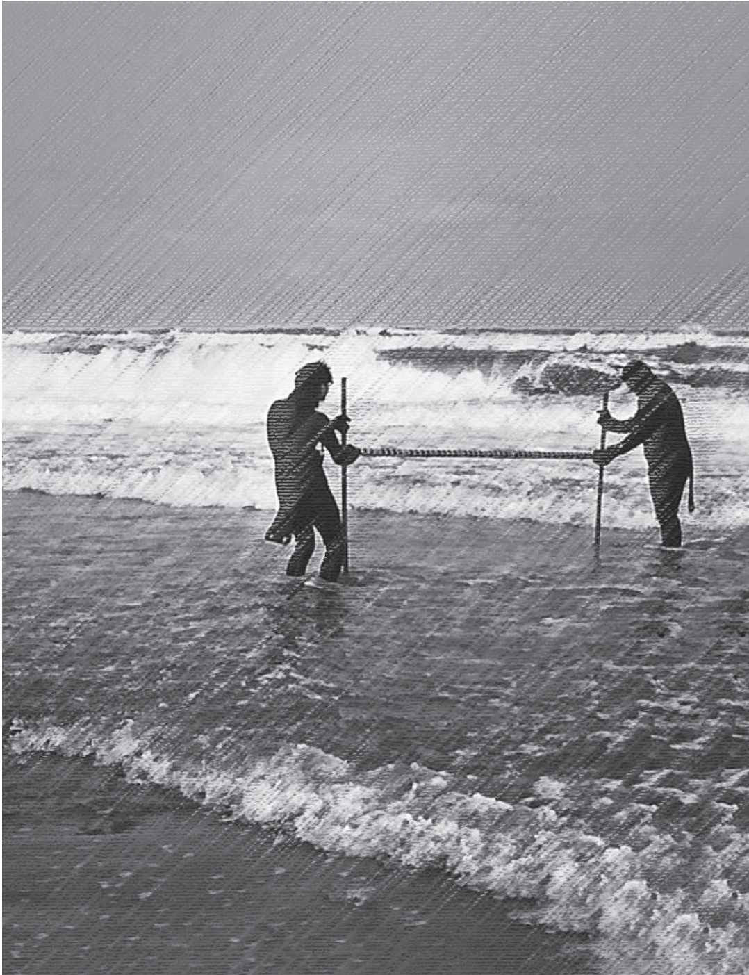
Coastal Heroes John Gifford and Walt Handy running a beach profile the old-fashioned way on Plum Island, Massachusetts, ca. 1969. These beach-profiling surveys, carried out at numerous locations between 1964 and 1972, allowed us to determine the beach erosional/depositional patterns for sand beaches along the northern New England coast.
