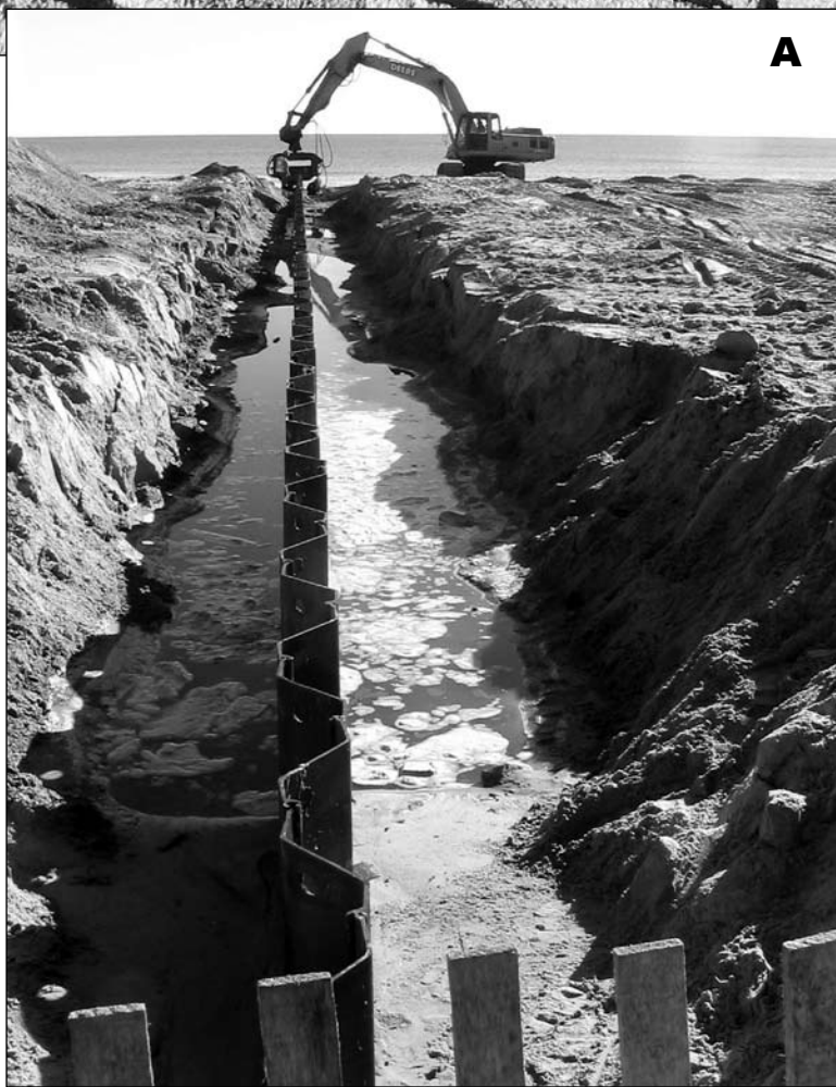
Figure 6. Construction photos of the groin installation project in January-February 2007. Steel sheet piles (20-ft long) were driven into the sand, following the natural profile of the beach (A and B). Armor stone was used for toe protection (C). Groin 2 at low tide in March 2007 (D).
