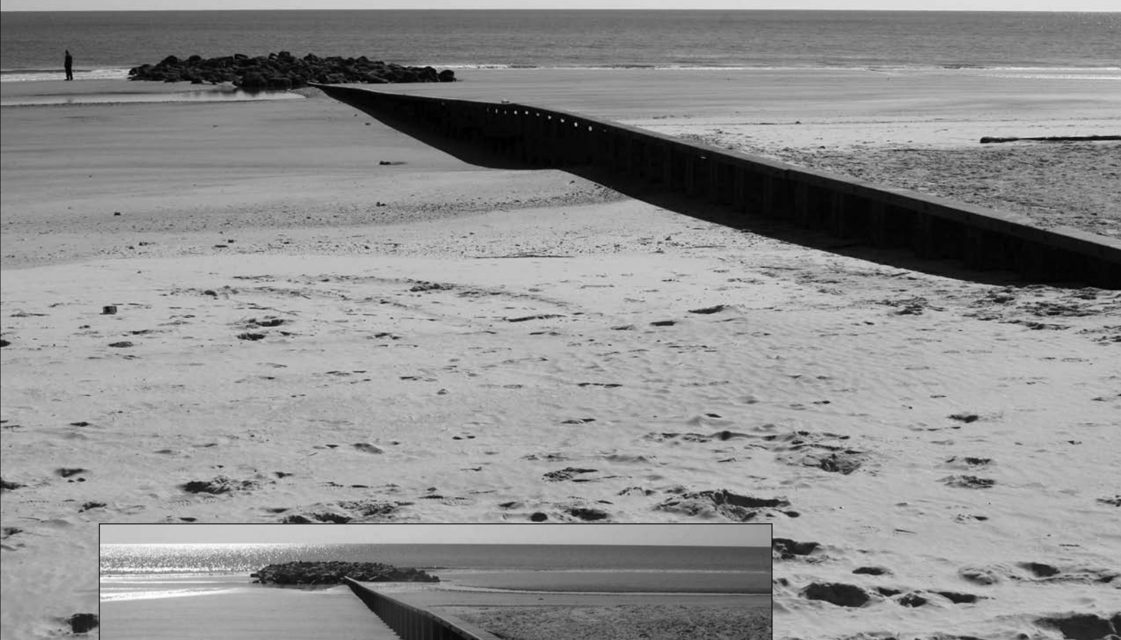
Figure 11. Post-project (April 2007) and January 2009 images of Groin 4 (upper) and Groin 7 (lower). All groins maintain a relatively low exposure (less than 4 ft), which was one of the goals of the project. “Template” groins, which slope to match the natural profile of the beach, are thought to maintain a lower reveal and offer better performance in the lower beach profile compared to most groins constructed in earlier decades, which often had little slope and terminated landward of the low-tide line.
