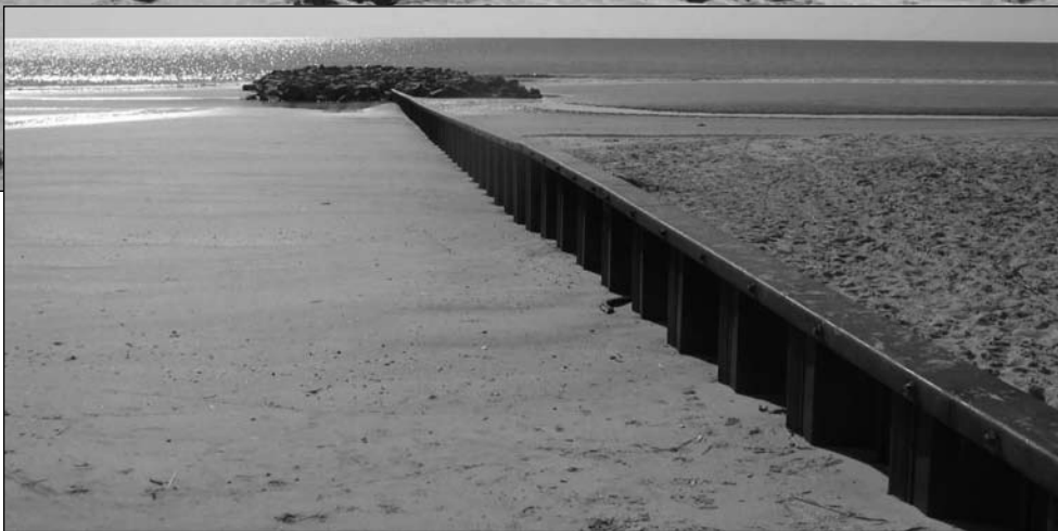
Figure 11. Post-project (April 2007) and January 2009 images of Groin 4 (upper) and Groin 7 (lower). All groins maintain a relatively low exposure (less than 4 ft), which was one of the goals of the project. “Template” groins, which slope to match the natural profile of the beach, are thought to maintain a lower reveal and offer better performance in the lower beach profile compared to most groins constructed in earlier decades, which often had little slope and terminated landward of the low-tide line.
