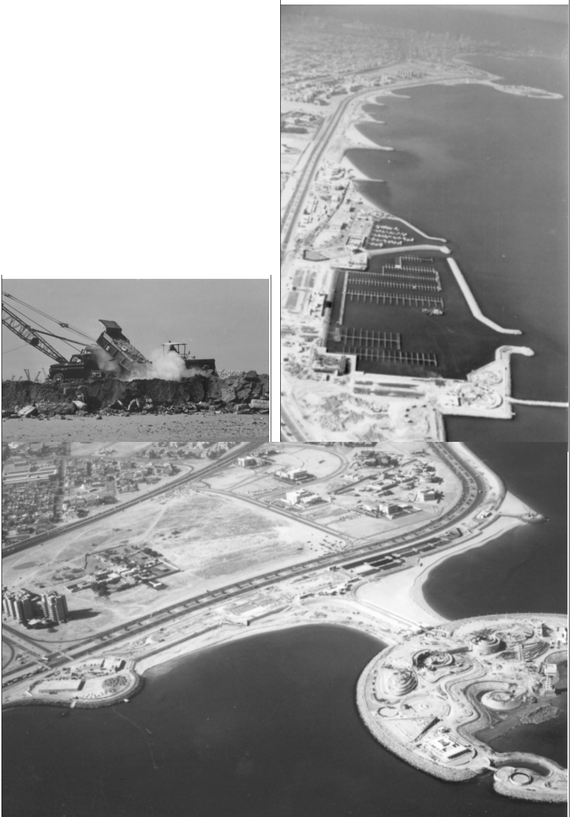
FIGURE 1. The Kuwait Waterfront Project involved restoration of beaches, construction of marinas, a “tombolo” island, and other park features along a 20-kilometer shoreline fronting Kuwait Bay. Early reclamation practice had degraded the shoreline by dumping debris. Photos by the author.
