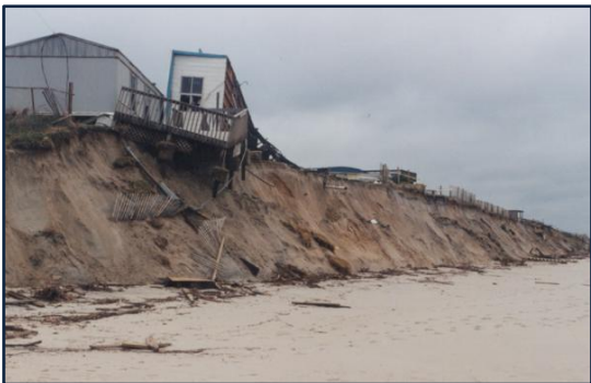
Indian Beach NC USA—After Hurricane Floyd (1999)—top of escarpment is >20 ft above MSL
